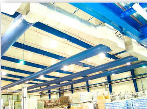
DuctSox products were initially developed exclusively for use in the food processing industry. The flexible fabric is a cost effective alternative to insulated stainless steel ducting and diffusers. Draft-free airflow through the woven fabric improves comfort for employees and reduces dehydration in the end product.
